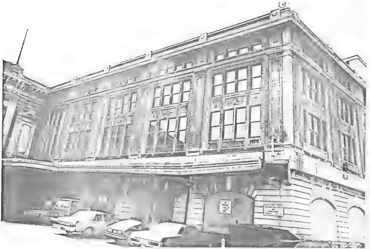
East and north facades of YMCA Building as viewed from ferry plaza. This building was constructed in two phases--the ground floor, with its rusticated arches, was built in 1907 as a baggage building. Sometime after World War I, the upper stories were added for a YMCA to serve trainmen (as designed, the baggage building's upper area was to be reserved for future office space). The upper stories of the building match the style of the 1907 terminal.
